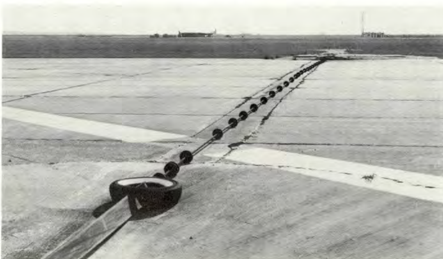
4. BAK-9 aircraft arresting barrier.
